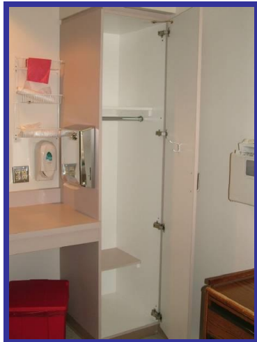
Hospital room closet before.
